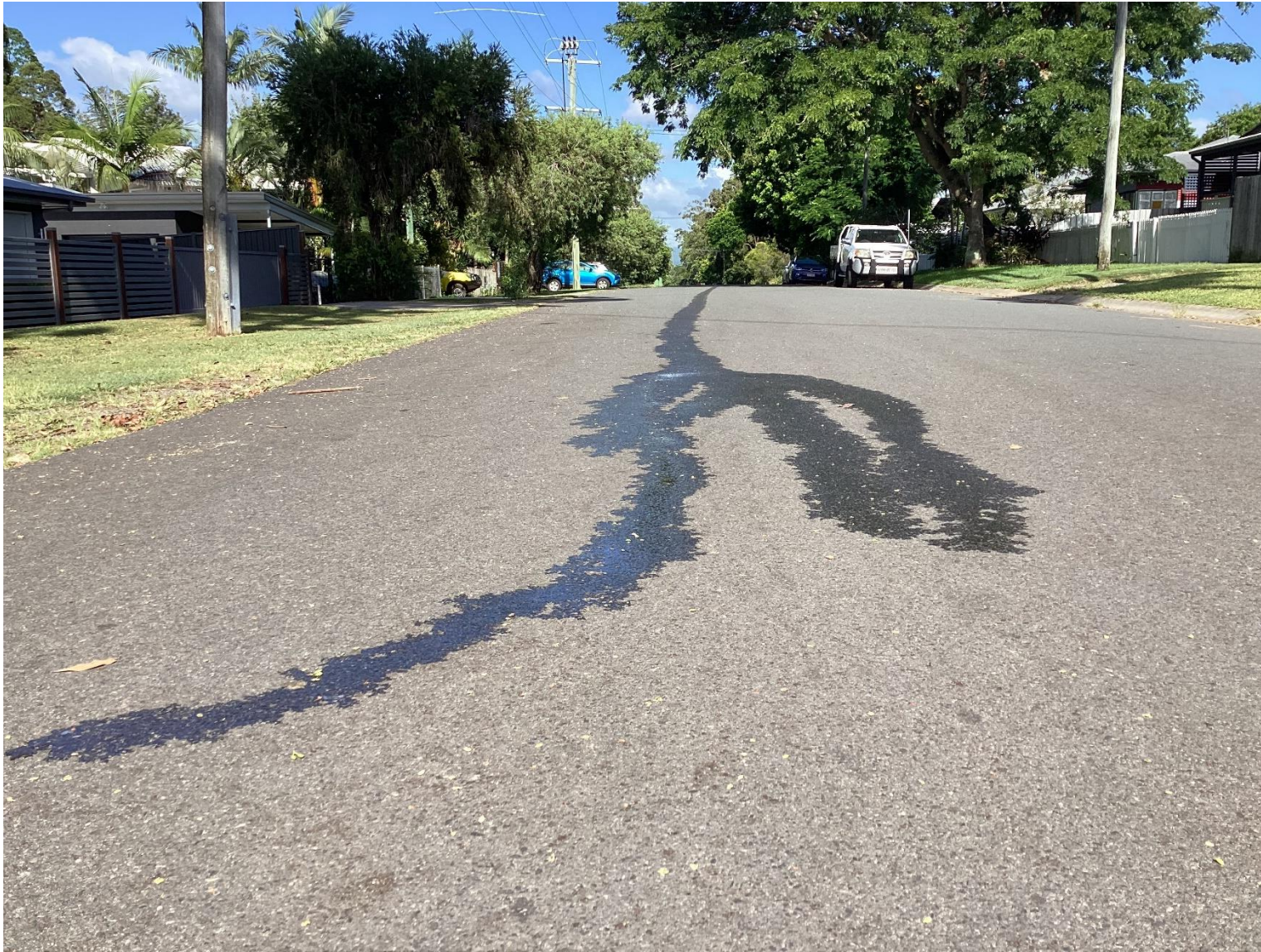
Figure 1. Van wastewater on Laguna St
